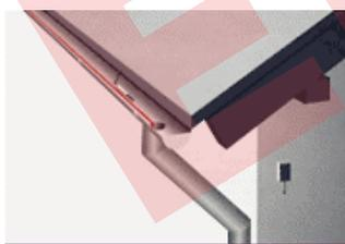
Thus, the heating power varies according to the temperature of the surface the heating tape is applied to.
